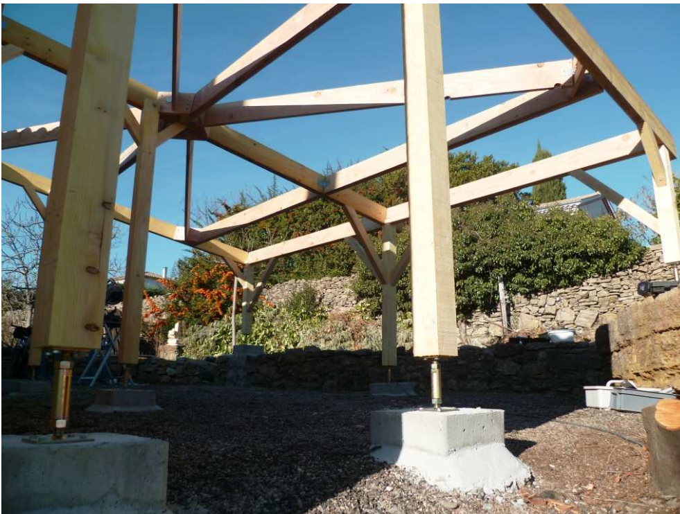
Structure porteuse (9 poteaux section 10/10cm)
